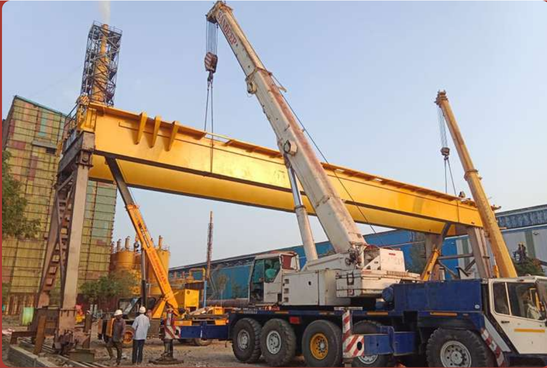
Major Refurbishment Erection Commissioning of 30 Ton x 32.4 x 70 M Goliath Gantry Crane of Major Steel Manufacturer at Pune
